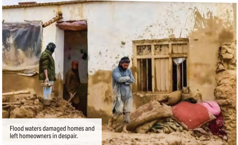
Afghani flood survivors look at the damage caused to their homes.
