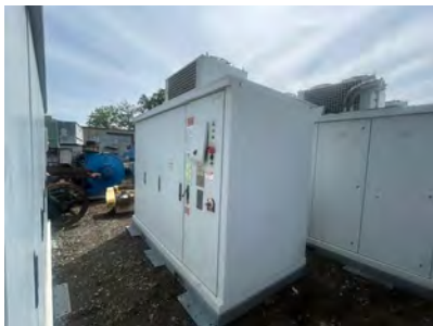
ABB Solar Inverters 3 Phase Solar Inverters Rated for Outdoor Use, INPUT 1000Vdc, Inverter Output 690Vac ULTRA-750-TL-OUTD-1-US-690-SSN4T-100000-0 Active Power 750-780kW $15,000.00 (1 Available) ULTRA-1100-TL-OUTD-1-US-690-SSN4T-100000-0 Active Power 1100 to 1170kW $20,000.00 (1 Available) ULTRA-1500-TL-OUTD-1-US-690-SSN4T-100000-0 Active Power 1500 to 1560kW $25,000.00 (2 Available)
