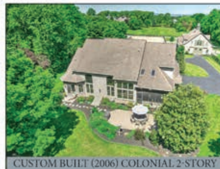
CUSTOM BUILT (2006) COLONIAL 2-STORY
