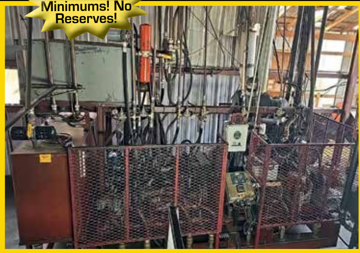
2009 Iveco Power Unit and Hydraulic Pack
