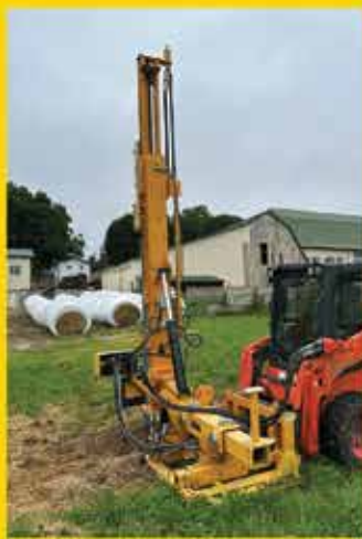
2022 Rhino Solar Pro Pile Driver Hillpoint, WI
