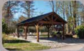
Pinecraft 16 x24 Timberframe Pavilion stained & installed with concrete floor.
