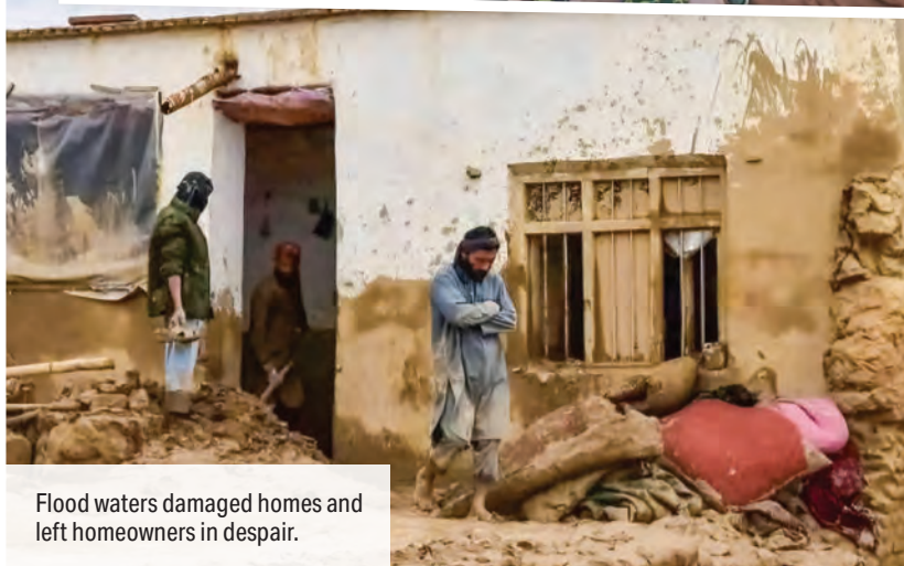
Afghani flood survivors look at the damage caused to their homes.
