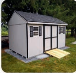
Showing 1 of 3 sheds!
