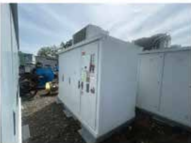
ABB Solar Inverters 3 Phase Solar Inverters Rated for Outdoor Use, INPUT 1000Vdc ,Inverter Output 690Vac ULTRA-750-TL-OUTD-1-US-690-SSN4T-100000-0 Active Power 750-780kW $15,000.00 ( 1 Available) ULTRA-1100-TL-OUTD-1-US-690-SSN4T-100000-0 Active Power 1100 to 1170kW $20,000.00 ( 1 Available) ULTRA-1500-TL-OUTD-1-US-690-SSN4T-100000-0 Active Power 1500 to 1580kW $25,000.00 ( 2 Available)
