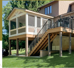
Second story balcony Done with fiberglass coating. Is roof for first story Screened in porch with open deck
