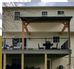
Second story balcony with fiberglass coating, serves as the roof for first story deck
