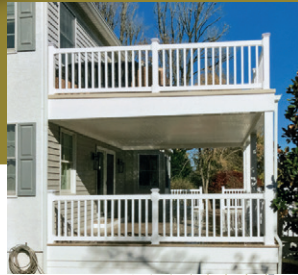
Second story balcony with fiberglass coating, serves as the roof for first story deck
