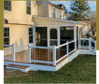
Screened in porch with open deck
